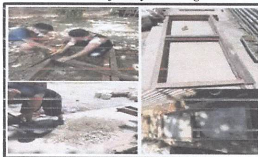
Figure 6. Preparation and making concrete slab
