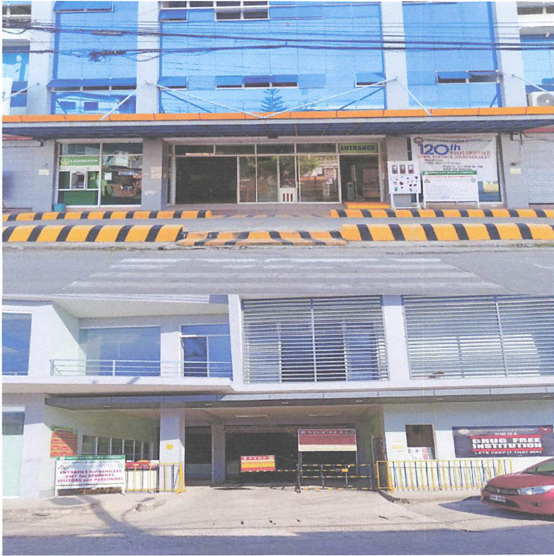
S.4. Entry and exit points permit the use of the building for public and other with minimum interference to school activities.
